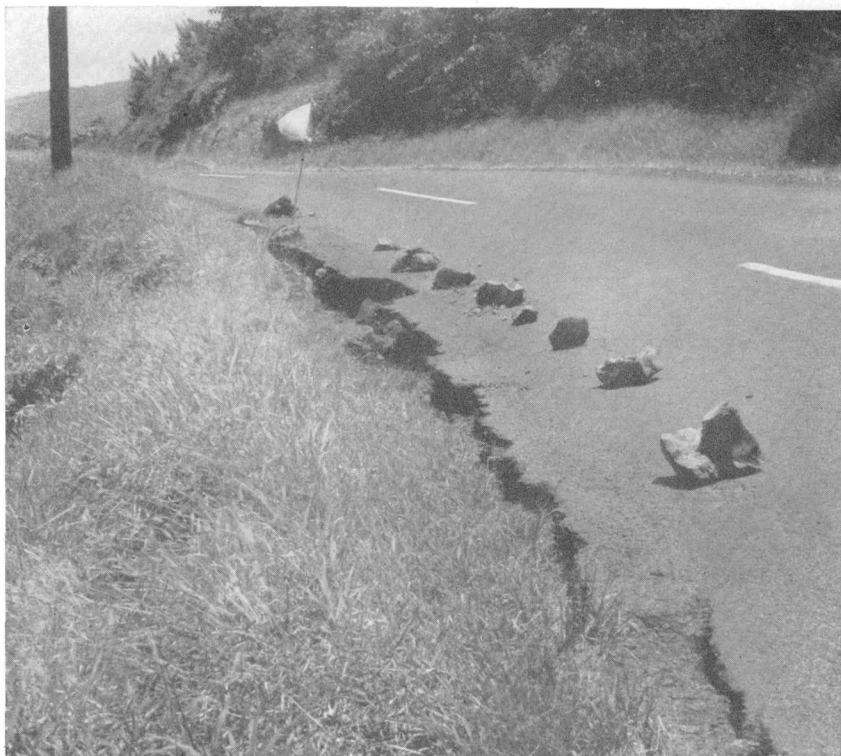
FIGURE 46.—Crack along the edge of the highway pavement 2 miles south from Kaimalino, apparently resulting from a downslope lurching of the shoulder, which moved as a separate unit from the part of the fill beneath the pavement.
