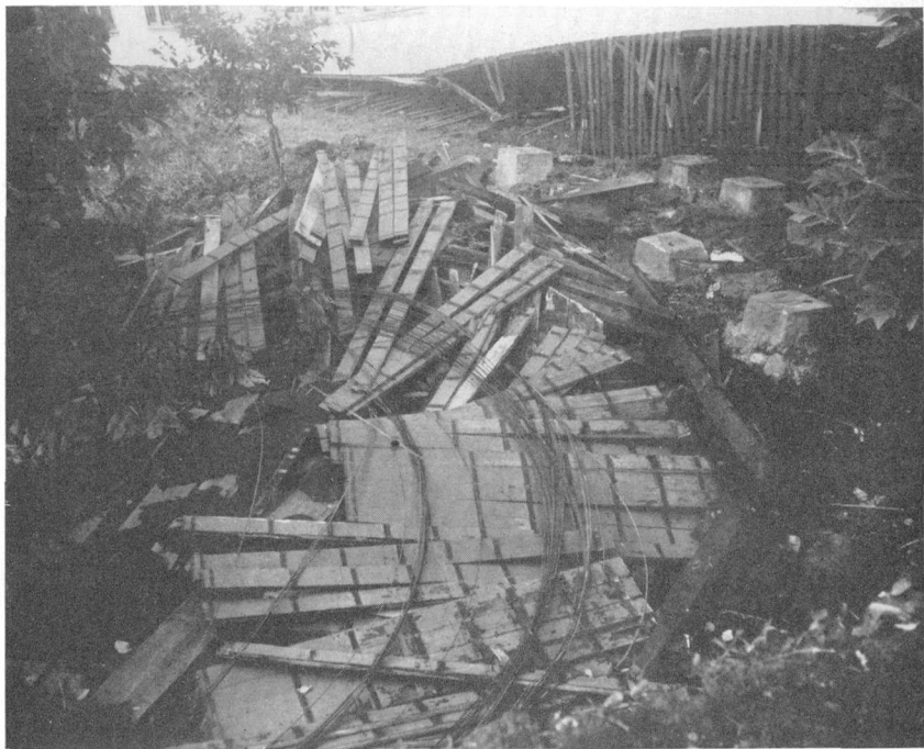
FIGURE 44.—Honaunau School building from the southwest. All but the south end of this building was dropped and moved westward owing to inadequate bracing of the underpinning in an east-west trending direction transverse to the longer dimension. The wood-stave water tank collapsed and was thrown westward from its concrete-block footings.
