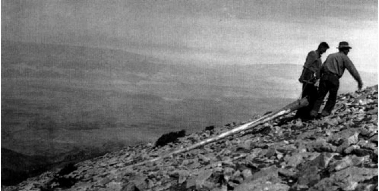
**Figure 10.** All in a day's work. C.B. Hunt and Charlie Hanks drag a heavy log of Engelmann spruce toward the summit of Mount Ellen, to be a pole for a triangulation flag. June 1936.
