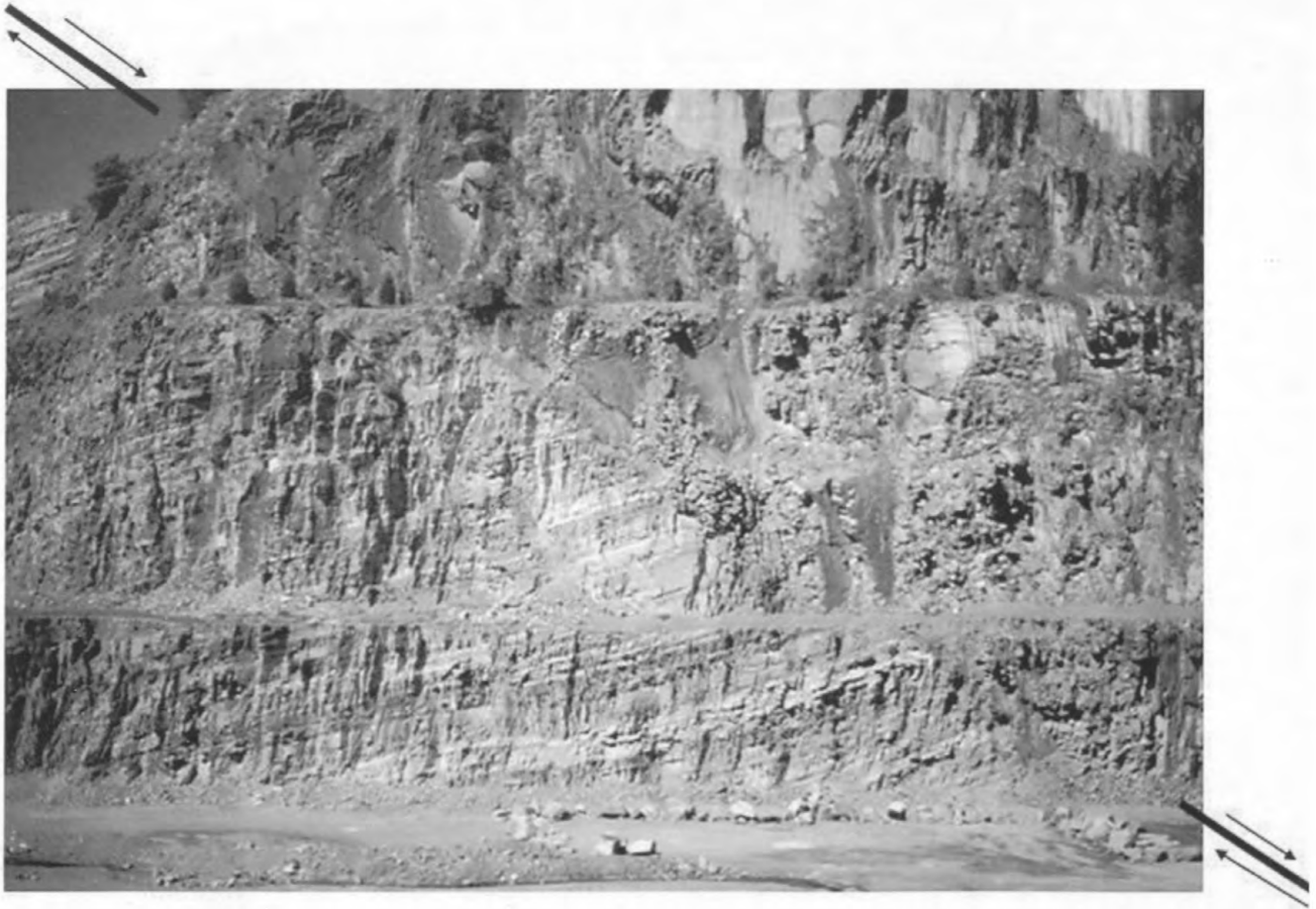
Figure 6. West-dipping Mesozoic strata cut by east-dipping normal fault (arrows) at Stop 6. Strata on east (right) side of fault are overlain by diabase sill and have dropped down relative to the west (left) side. Photograph faces north.
