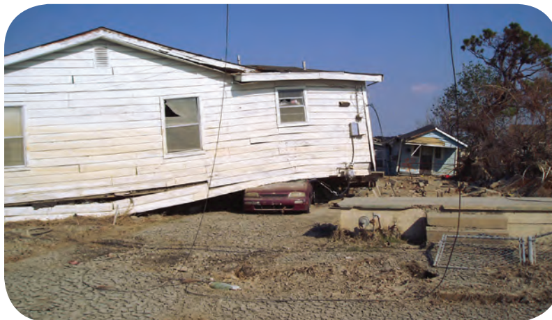
Figure 1. Photograph showing destruction of property and deposited sediment from flood waters in the Ninth Ward, New Orleans, La., after Hurricane Katrina in 2005.
