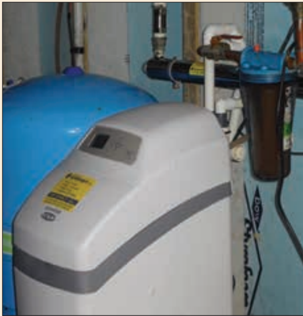
Example of domestic-well user's home water-treatment system.
