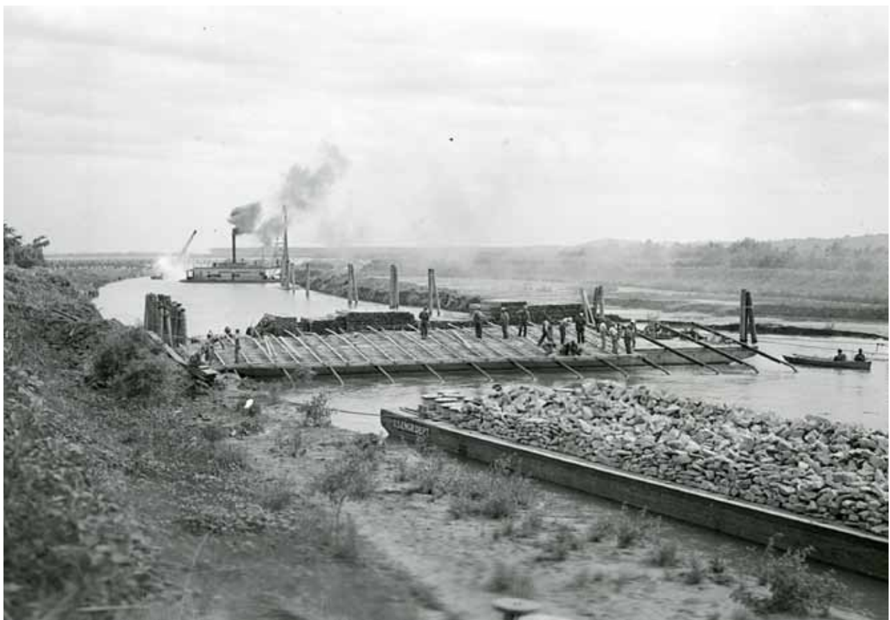
Figure 7. Construction of Missouri River revetment, June 2, 1938 (source: U.S. Army Corps of Engineers).
