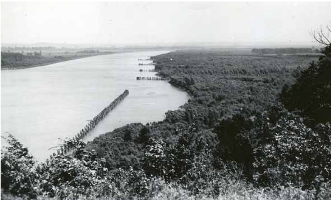
Figure 8. The siltation of a dike system, Indian Cave Bend, Missouri River (source: U.S. Army Corps of Engineers, Omaha District).—Continued
