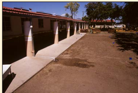
E. Daycare facility after remediation that included complete substrate removal. (Photo by William J. Murray)
