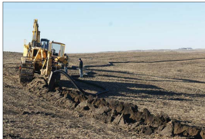
Drainage pipe being installed in wetland catchment. Photograph by Charles Dahl, U.S. Geological Survey.
