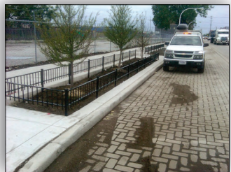
Permeable pavement Cermak-Blue Island Streetscapes Corridor. Photo by James Duncker, U.S. Geological Survey.
