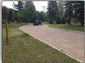
Orange Village Park permeable pavement parking lot. Source: Winston and others, 2015.
