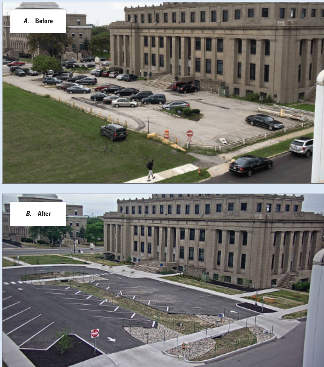
Figure S1.1. City Hall, Gary, Indiana, before and after installation of central rain garden and peripheral grassed areas.
