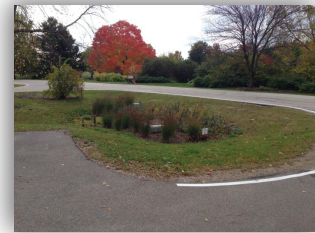
Holden Arboretum bioretention cell. Source: Winston and others, 2015.
