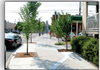
Tree trench examples in Harrisburg, Pennsylvania. Source: Capitol Region Water, 2017.
