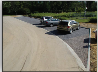
Old Woman Creek National Estuarine Research Reserve visitor center permeable interlocking concrete pavement. Source: Winston and others 2015.
