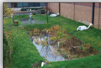
Madison Water Supply Pump House rain garden in clay soil. Source: Selbig and Balster, 2010.
