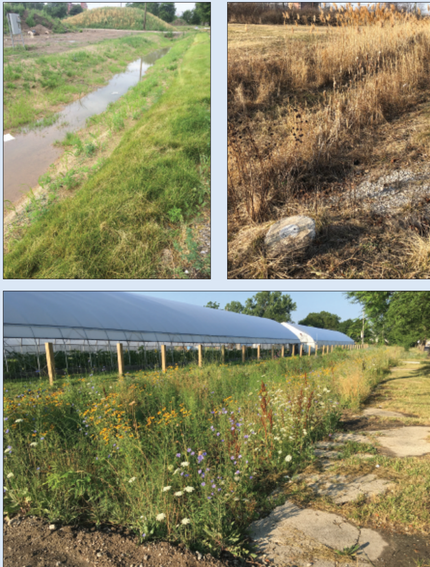
Figure S3.2. Vegetated swales and stormwater capture system installed in RecoveryPark, Detroit, Michigan. (Courtesy of U.S. Geological Survey).
