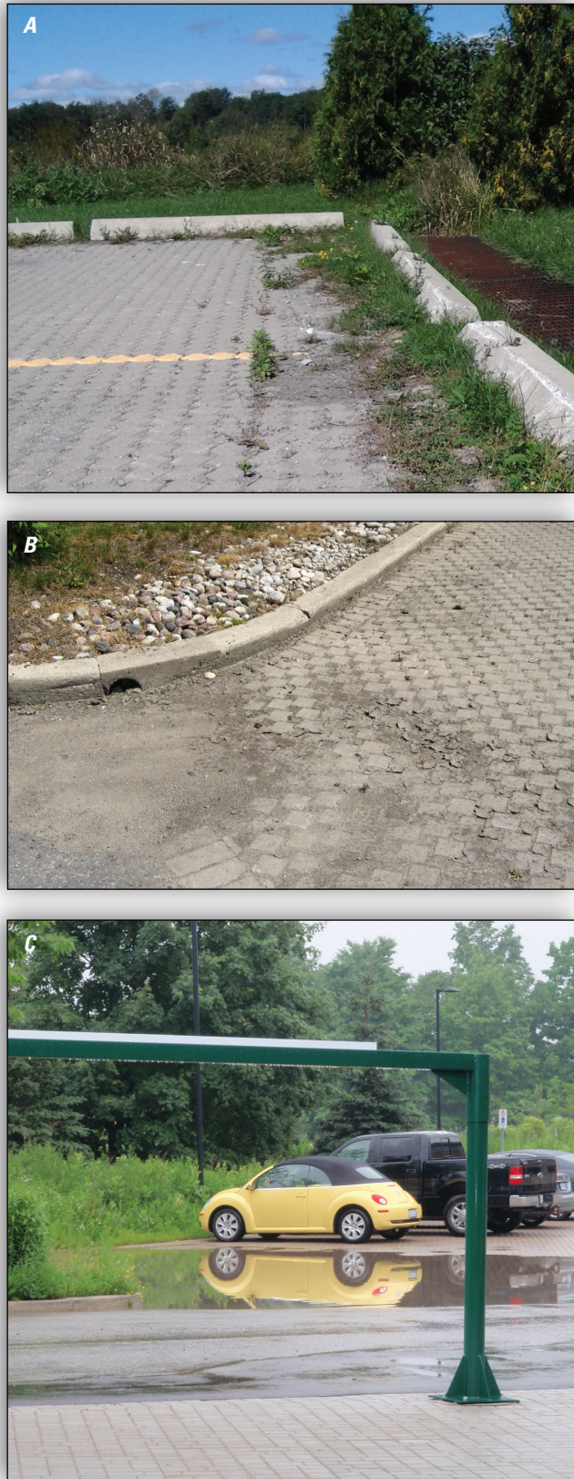
Figure 29. Examples of permeable pavement systems showing accumulation of sediments (A and B) and partial infiltration (C). (Source: Sustainable Technologies Evaluation Program, 2018.)
