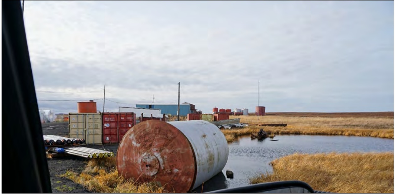
Storage tank overturned because of flooding in western Alaska. Photograph by Ryan Toohey, Alaska Climate Adaptation Science Center.
