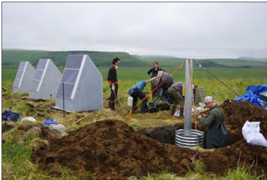
Installing the Very Small Aperture Terminal (satellite communications node) at Fort Glenn, Alaska, on the eastern flank of Okmok caldera as part of the 2021 Analog to Digital campaign. Photograph by Pavel Izbekov, U.S. Geological Survey and University of Alaska Fairbanks Geophysical Institute.
