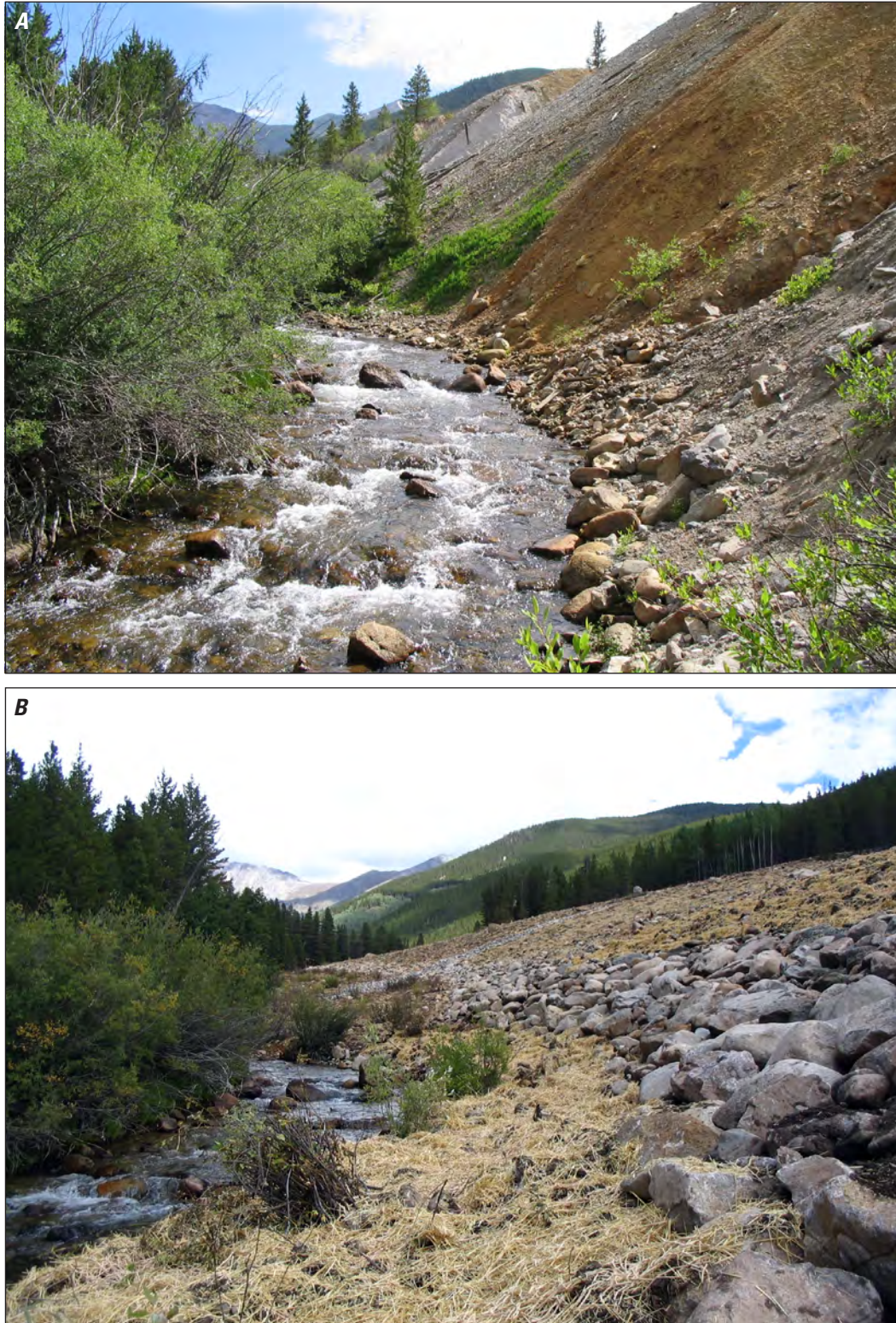
Figure 2. The Akron Mine and Mill Site is an abandoned mine and ore processing site near Whitepine, Colorado, that was active from 1885 to 1893. A , Waste rock and tailings in direct contact with Tomichi Creek [Photograph by U.S. Department of Agriculture Forest Service Rocky Mountain Region]. B , Restoration actions that were completed in August 2016 that removed waste material away from the creek and restored the affected channel and floodplain [Photograph by U.S. Department of Agriculture Forest Service Rocky Mountain Region].
