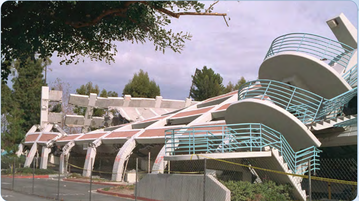
Northridge parking garage as a result of the January 17, 1994, magnitude 6.7 Northridge, California, earthquake. Photograph by U.S. Geological Survey.
