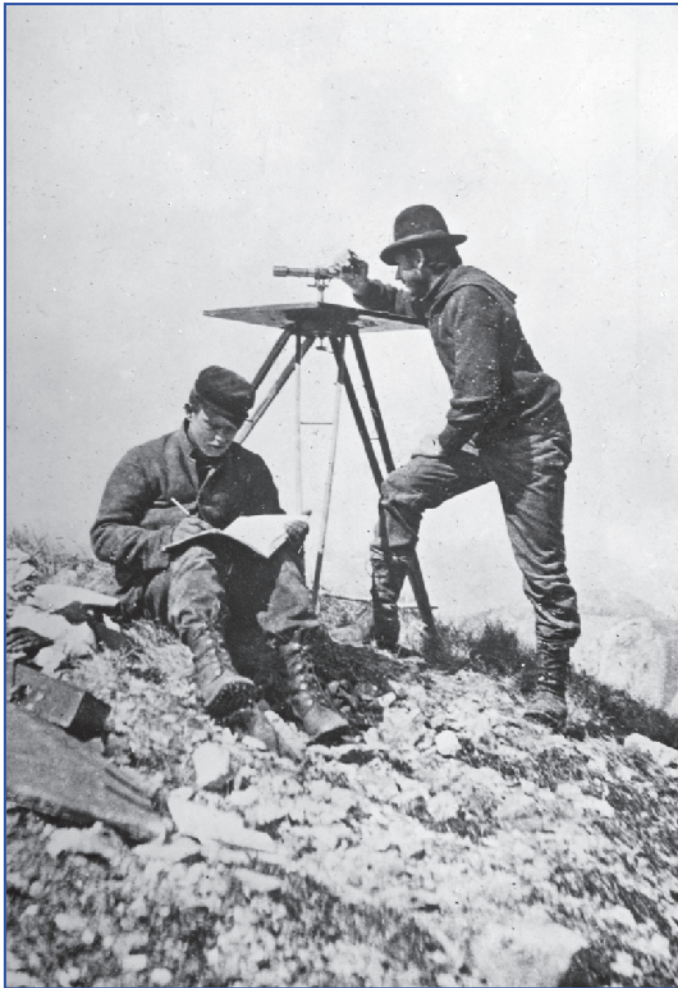
Figure 20. Photograph illustrating the use of a plane table and telescopic alidade, Canadian boundary, circa 1906. Photograph appears courtesy of U.S. Geological Survey Denver Library Photographic Collection.
