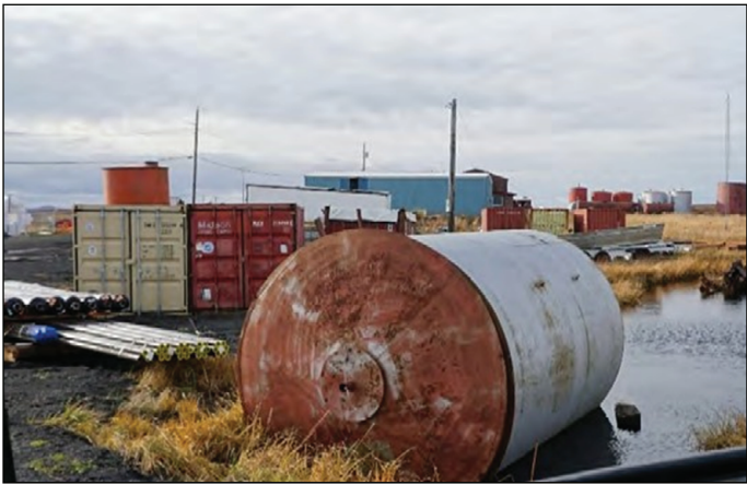
Photograph showing a storage tank overturned because of flooding in western Alaska. Photograph by Ryan Toohey, U.S. Geological Survey.
