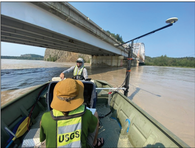
Photograph showing U.S. Geological Survey staff doing a multibeam and lidar survey at Tanana River at Big Delta, Alaska, to access scour conditions at the Richardson Highway Bridge in July 2023. Photograph by Hiram Henry, Alaska Department of Transportation and Public Facilities.
