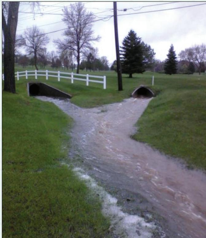
**Figure 4.** Photograph showing stormwater runoff through culverts in the Arrowhead drainage basin immediately below Arrowhead Country Club during a May 2010 storm event in Rapid City, South Dakota. Runoff from this drainage discharges into Rapid Creek. Photograph by Galen Hoogestraat, U.S. Geological Survey.
