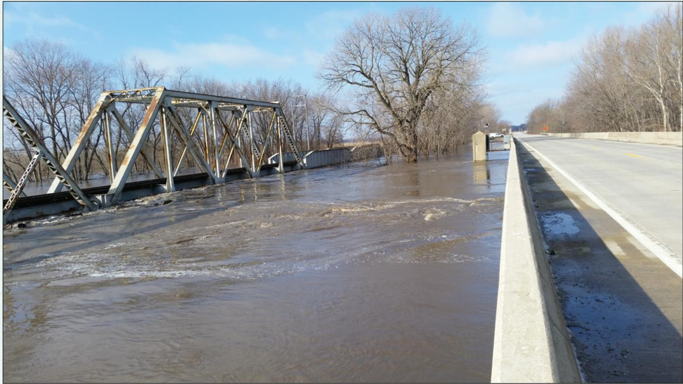
**Figure 9.** Photograph showing flooding conditions at U.S. Geological Survey streamgage 05583000 (Sangamon River near Oakford, Illinois) on January 1, 2016. Daily mean streamflow on this date was measured as 71,700 cubic feet per second. Photograph by Perry Draper, U.S. Geological Survey.
