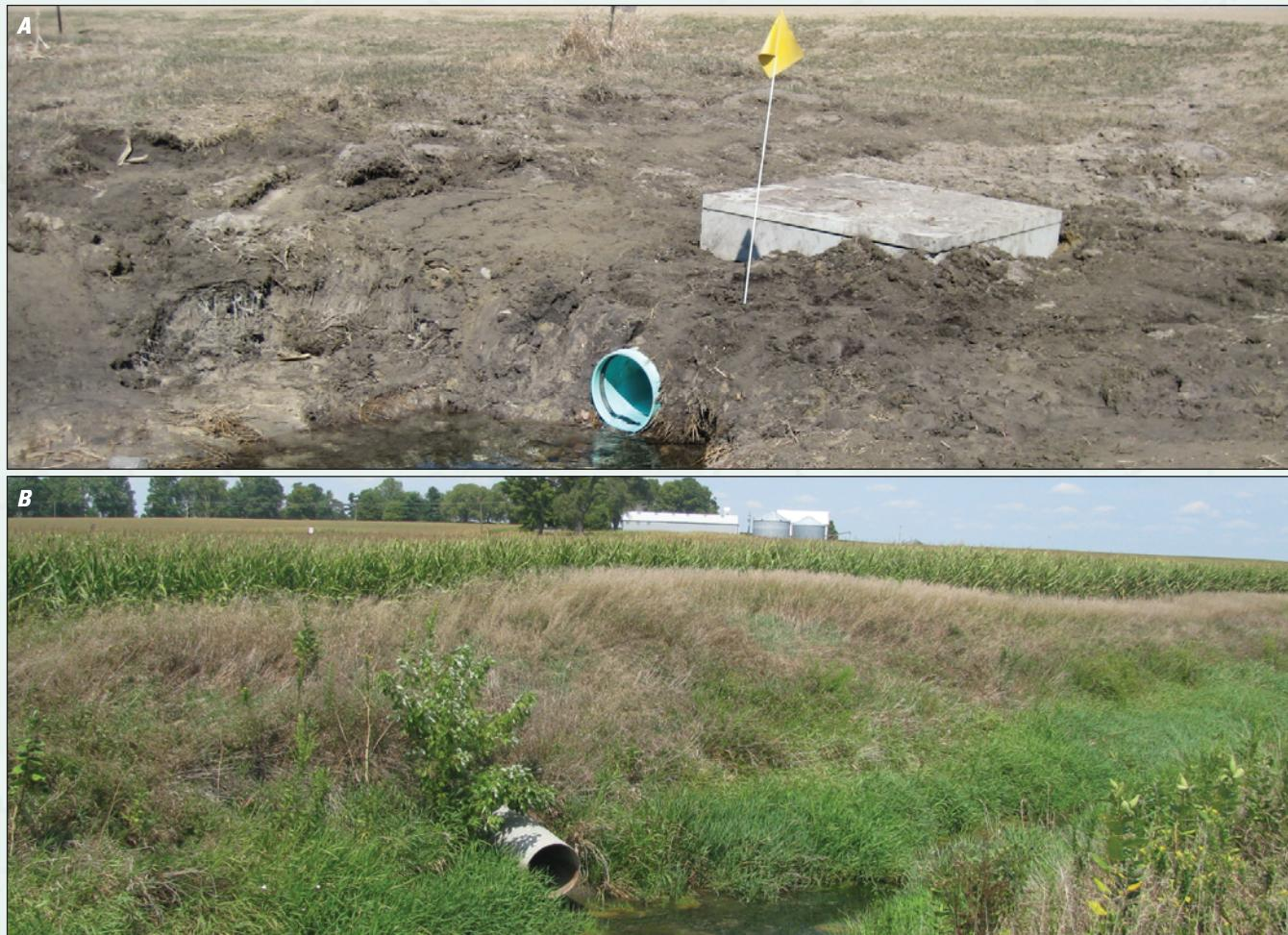
**Figure 40.** Photographs showing subsurface agricultural tile drainage outlets (A) near Embden, North Dakota, and (B) in the Midwestern Corn Belt. Photographs by (A) Kathleen Rowland and (B) Peter Van Metre, U.S. Geological Survey.
