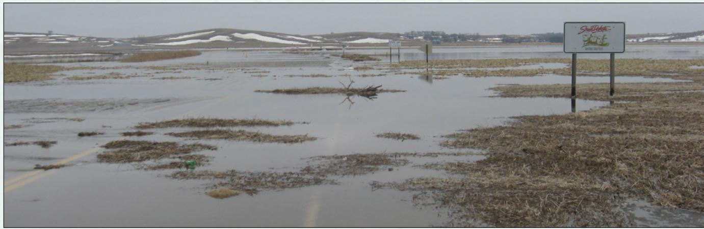
**Figure 12.** Photograph showing flooding conditions at U.S. Geological Survey streamgage 06485500 (Big Sioux River at Akron, Iowa) on March 17, 2010. Daily mean streamflow on this date was more than 30,000 cubic feet per second. Photograph by Nate Stevens, U.S. Geological Survey.
