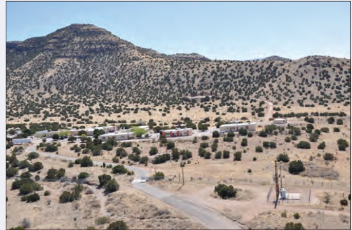
Figure 1. Photograph of the Albuquerque Seismological Laboratory taken from Kirtland Air Force Base looking south toward the lab. The underground vaults are on the side of the hill in the back. This location was selected for being an exceptionally low-noise site. Photograph by the U.S. Air Force.
