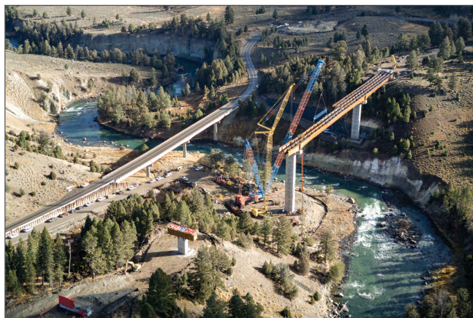
Figure 3. Yellowstone River bridge replacement project near Tower Junction, Wyoming. The existing bridge span, at the left, will be removed and the road realigned when the new bridge span, under construction to the right, is completed. Photograph by Jacob Frank, National Park Service, October 24, 2024.
