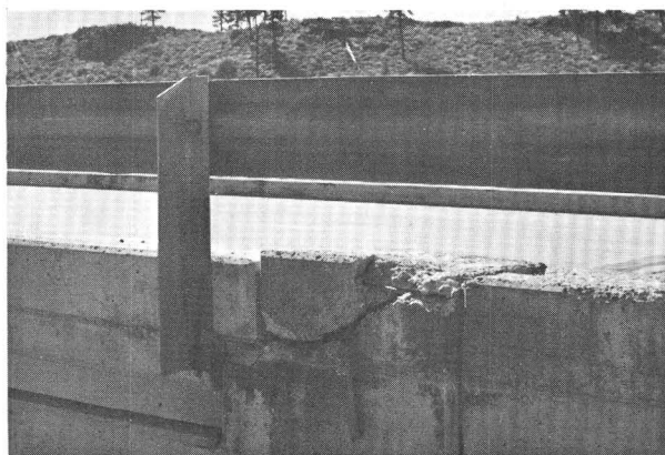
FIGURE 7.—Damage to east abutment of eastbound lane bridge on Interstate Highway 80 where it spans railroad tracks and Truckee River at Union Mills. View to the northeast.
