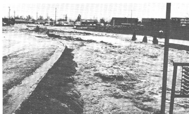
Figure 3.—Effect of coarse-sediment deposition on flow capacity in urban channels. A , Flow of sediment in floodwater from the January 1969 storms plugged a Glendora, Calif., concrete-lined channel and caused overflow and deposition on nearby property. The channel had been partly cleaned after the flood and before the picture was taken. B , Three feet of deposition in the lower part of this boulevard channel in Boulder, Colo., caused flooding by a flow of less than one-fifth the design capacity of the channel.
