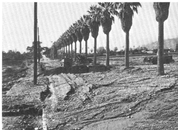
Figure 5.—More than 1,000 cubic yards of debris deposited on a short section of Ledora Avenue, Glendora, Calif., during the January 1969 storms by sediment flow and floodflow from nearby recently burned foothill area.
