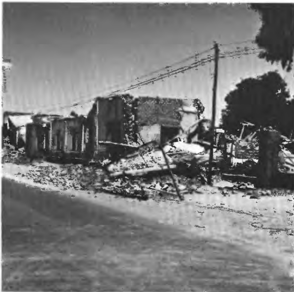
Figure 13.- Collapsed one-story adobe dwellings in Caucete, 80 km southwest of epicenter. Tilted streetlight in background was pulled over when face of adjacent building collapsed on wires suspended between poles.
