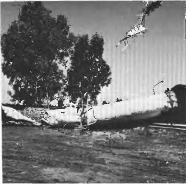
Figure 10.- Collapsed wine storage tank at Covic Winery in Media Agua, 117 km southwest of epicenter. Vertical steel anchor ties at base pulled loose as a result of rocking action of tank.
