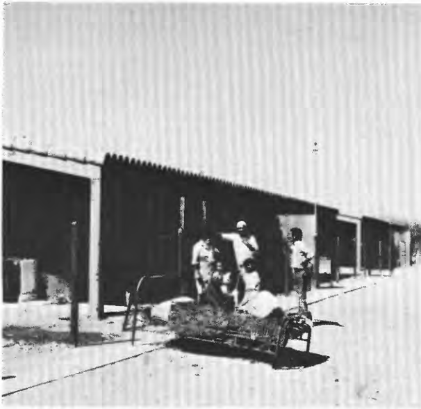
Figure 12.- Undamaged recently constructed reinforced masonry dwellings in Bermejo, 55 km south of epicenter. Nearby unreinforced masonry and adobe buildings partially or totally collapsed.
