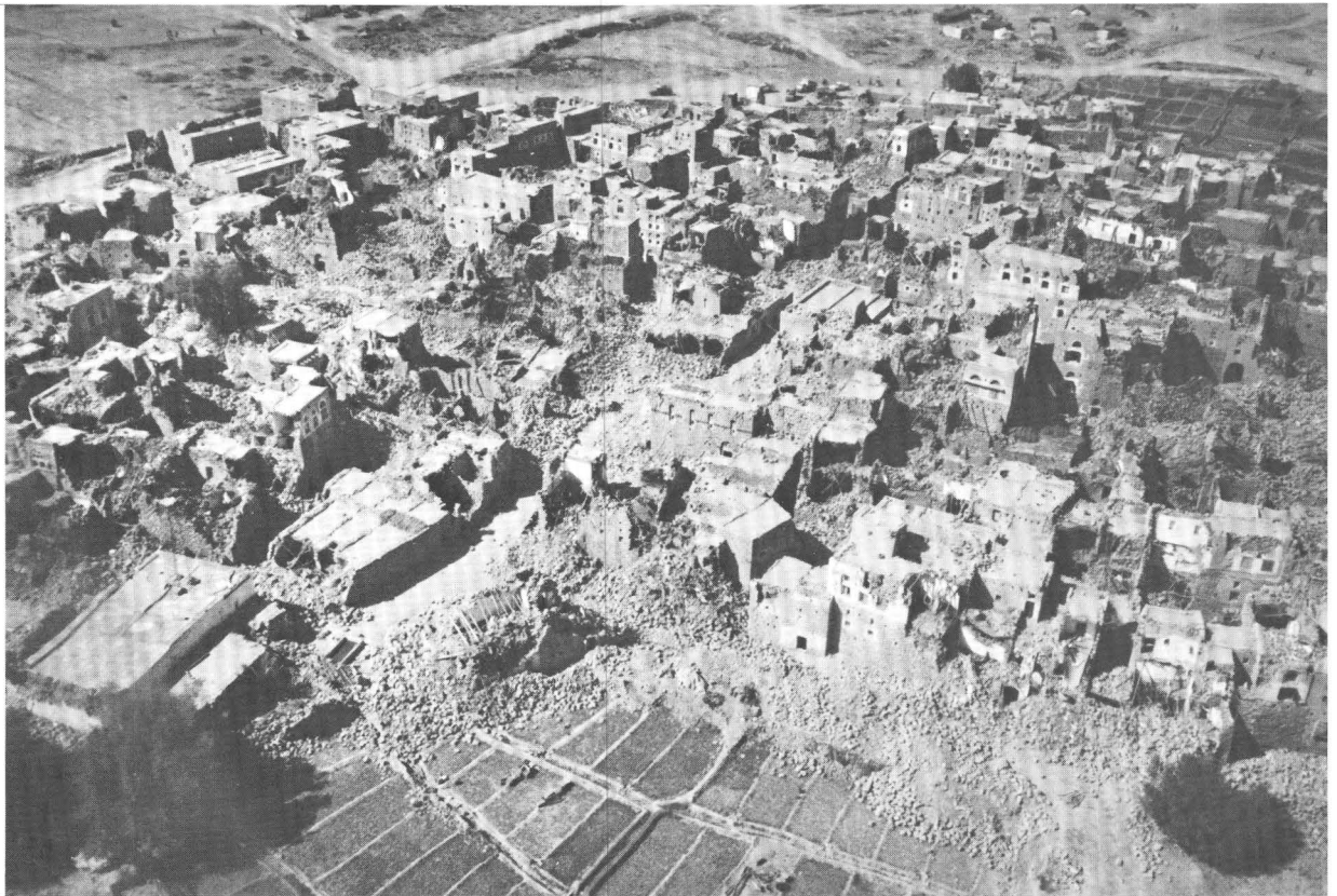
Much of the unreinforced stone masonry in Risabah, Yemen, collapsed during the December 13, 1982, earthquake. The city was approximately 6 miles from the epicenter of the magnitude 6.0 shock.
