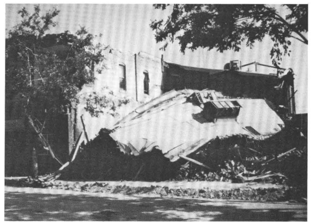
Destruction of unreinforced masonry buildings, showing wall failure and collapse of top stories, during the Coalinga earthquake of May 1983.
