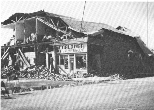
Destruction of unreinforced masonry buildings, showing wall failure and collapse of top stories, during the Coalinga earthquake of May 1983.
