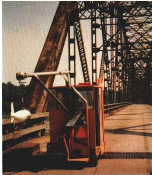
Suspended-sediment samples were collected from the Mississippi River at Chester, Illinois, by using a US P-63 sampler suspended from a specially designed boom-hoist car.
