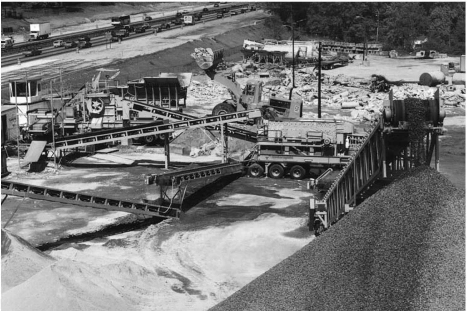
Figure 13. Typical recycled aggregates operation. (Courtesy of Cedarapids.)
