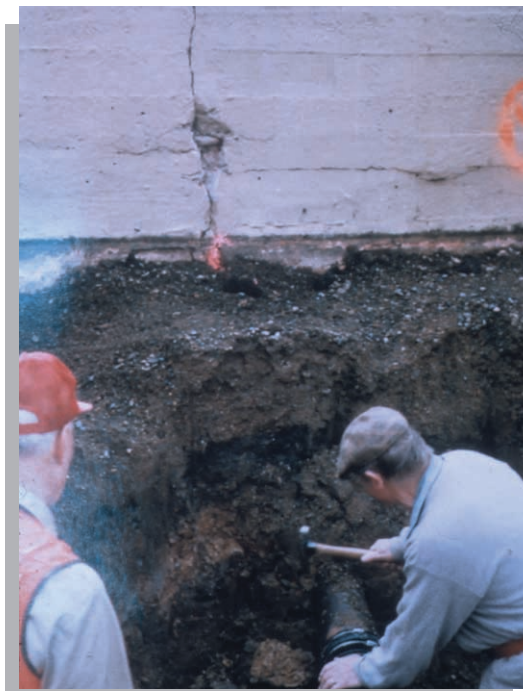
Geologists studying earthquake effects on and beneath a bridge.
