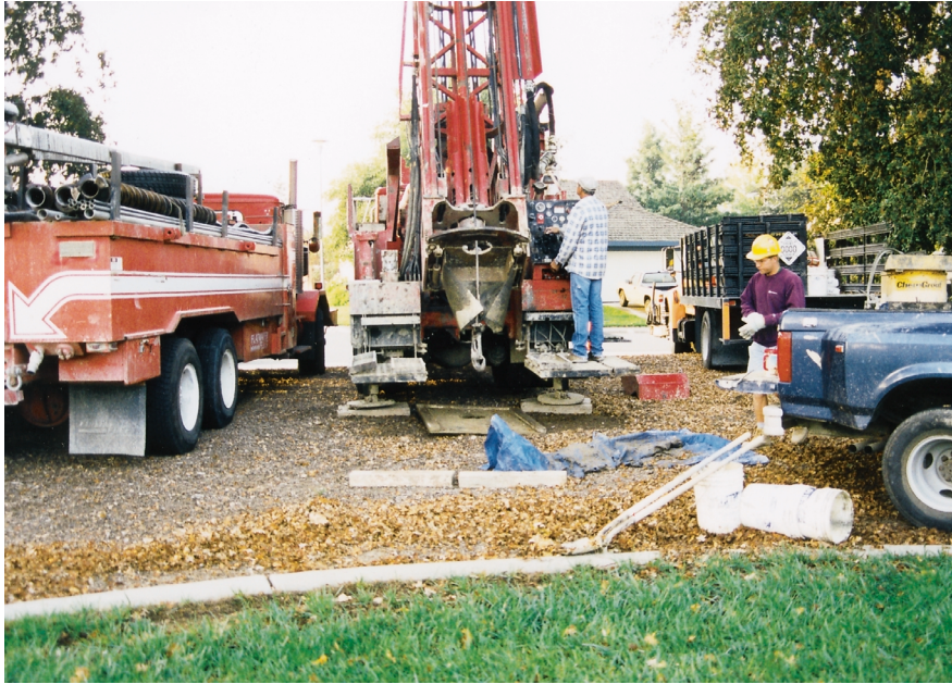
Figure 21. Drilling and installation of a new monitoring well in the Sacramento metropolitan area. This study of shallow ground water was the first of its kind within the Sacramento metropolitan area.
