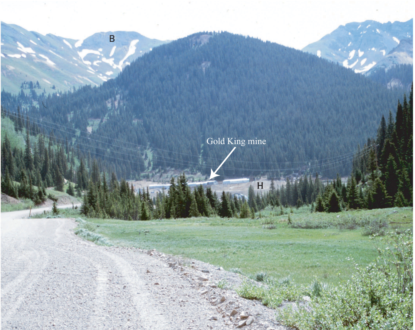
2. Human works (H). Looking north and northeast along Cement Creek toward Gold King mine at Gladstone. Arrow also is near the recent American Tunnel adit access to the Sunnyside mine. Mines are inactive since 1992 but reclamation activities are presently taking place. Slopes are mostly forest-covered colluvium (c), not visible at this scale, and bedrock (B).
