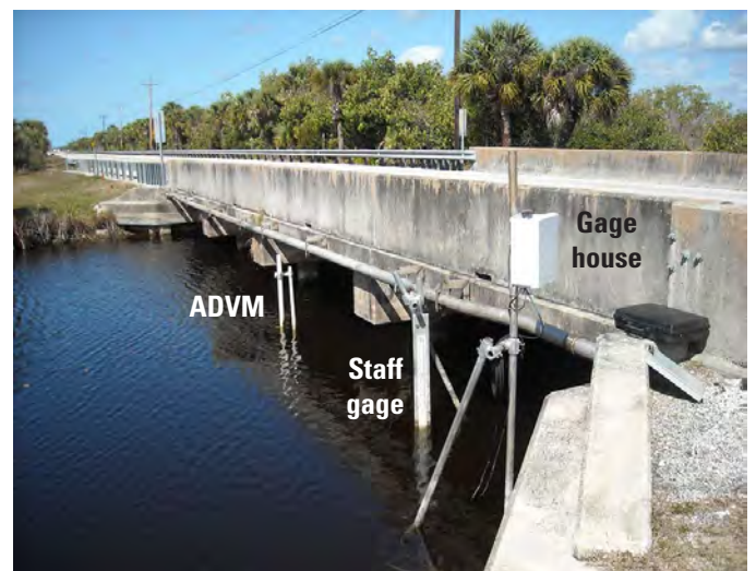
Figure 3. Index velocity station at Bridge 55 (photograph by Lars Soderqvist, U.S. Geological Survey).
