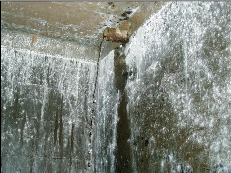
**Figure 14.** Inflow to the cistern at Split Rock Spring through 2-inch diameter steel pipe near the cistern ceiling.
