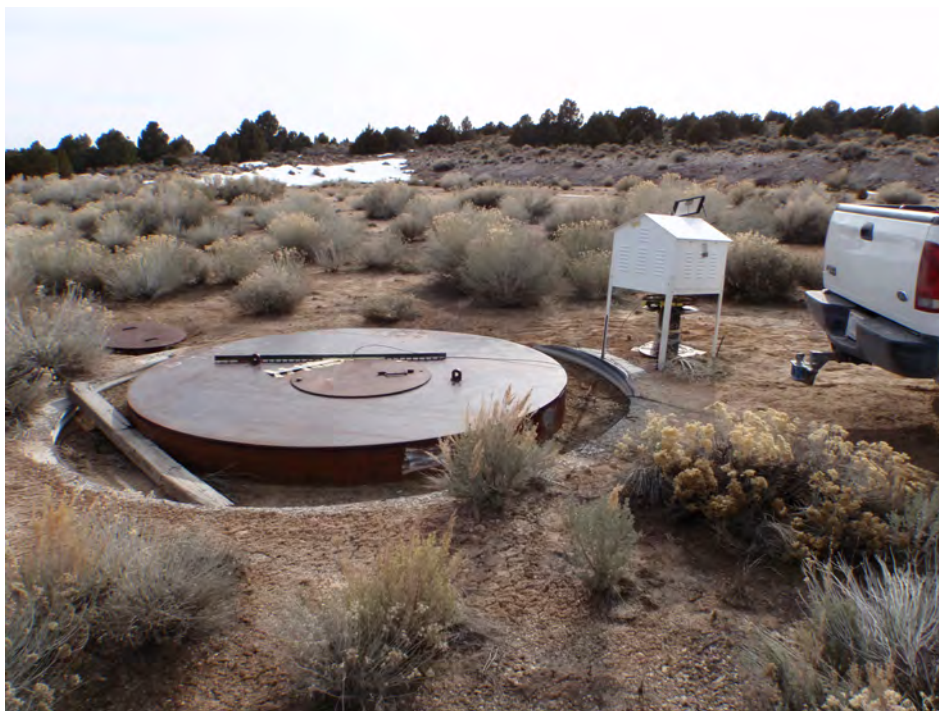
Figure 14. View facing west of U-20bg monitoring hole on Pahute Mesa, Nye County, Nevada. Snow-covered scarp created from construction of drill pad. Corrugated metal pipe surface casing is 136-inch diameter to 8 feet. Conductor casing is 122-inch to 57 feet. 96-inch-diameter open hole to a total depth of 2,200 feet. (Photograph taken by Steven R. Reiner, U.S. Geological Survey.)
