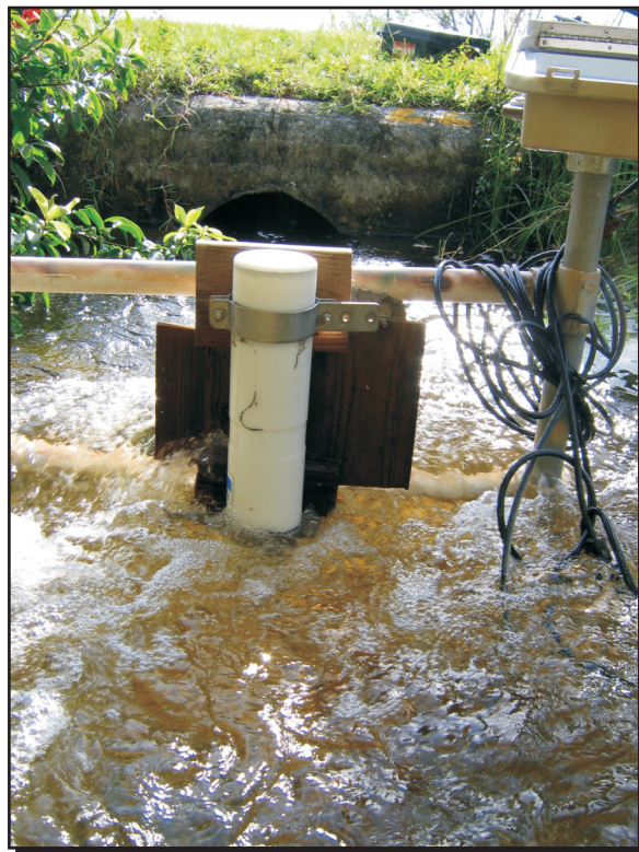
Figure 9. High-flow velocity that exceeded the Argonaut-ADV® program setting, causing suspect data spikes. Suspect data were deleted from this study.
