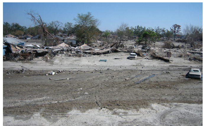
Figure 1. Levee breach damage in the Lower Ninth Ward of New Orleans along the Inner Harbor Navigational Canal (IHNC).
