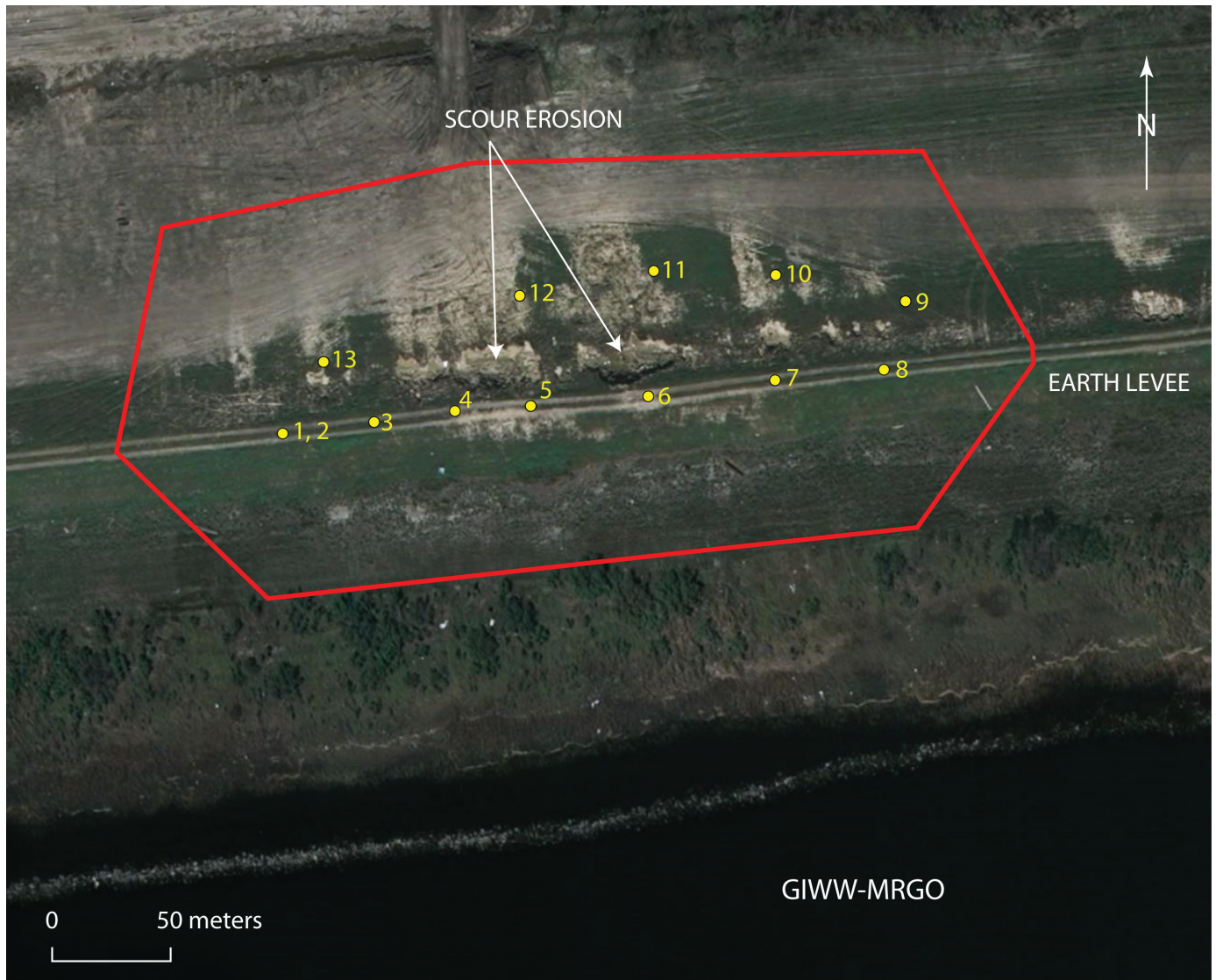
Figure 13. Site 7—Gulf Intracoastal Waterway–Mississippi River Gulf Outlet (GIWW-MRGO) earth levee erosion. Numbered dots indicate locations of scan positions. Red outline indicates area of lidar data coverage. (Photo source: Google Earth–USGS image.)
