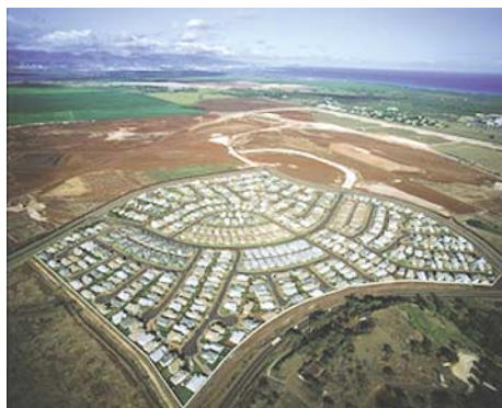
Central Oahu--an area of rapidly changing agricultural and suburban land use. The area is underlain by the island's principal drinking-water aquifer, part of which is designated a "sole source aquifer" by the USEPA in 1987 (photo by Douglas Peebles).
