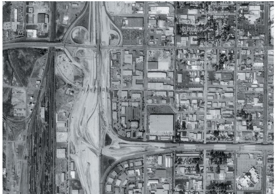
Figure 4. Aerial photograph of an urban interchange under construction
