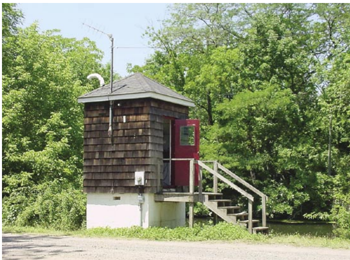
Figure 2. Typical "real-time" surface-water gaging station equipped with a data-collection platform and satellite antenna.
