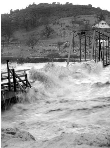
Figure 2. Flood waters washing out bridge.
