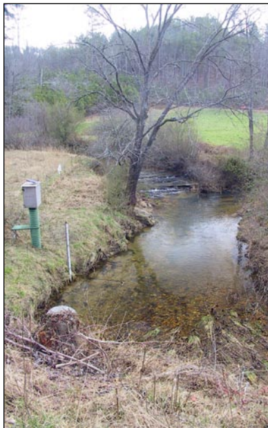
A streamflow monitoring station (middle left) measures water level of a stream; from this, streamflow can be computed.
