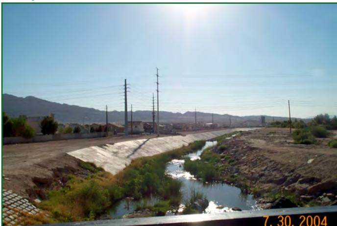
Las Vegas Wash looking downstream.
