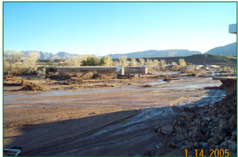
Figure 4. View of flood damage along Beaver Dam Wash at Beaver Dam, AZ, January 14, 2005.
