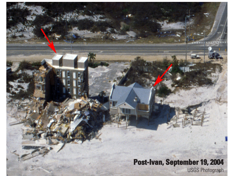
Figure 2. Orange Beach, Alabama. USGS aerial photographs taken before and after the landfall of Hurricane Ivan show the failure of a five-story condominium tower. The only parts of the structure that remain standing after Hurricane Ivan are the elevator and stairwell shafts. Airborne laser mapping data showed that the sand dune on which this building was constructed was subjected to about 3 m of vertical erosion during the storm. (Arrows in all images point to the same feature.)
