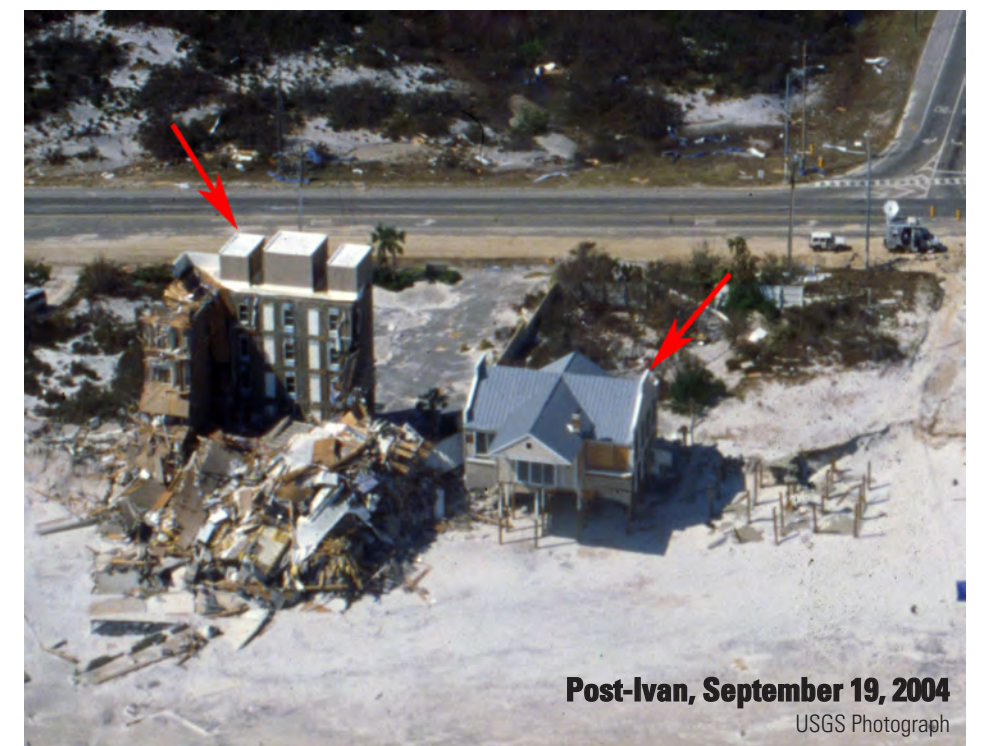
Figure 2. Orange Beach, Alabama. USGS aerial photographs taken before and after the landfall of Hurricane Ivan show the failure of a five-story condominium tower. The only parts of the structure that remain standing after Hurricane Ivan are the elevator and stairwell shafts. Airborne laser mapping data showed that the sand dune on which this building was constructed was subjected to about 3 m of vertical erosion during the storm. (Arrows in all images point to the same feature.)
