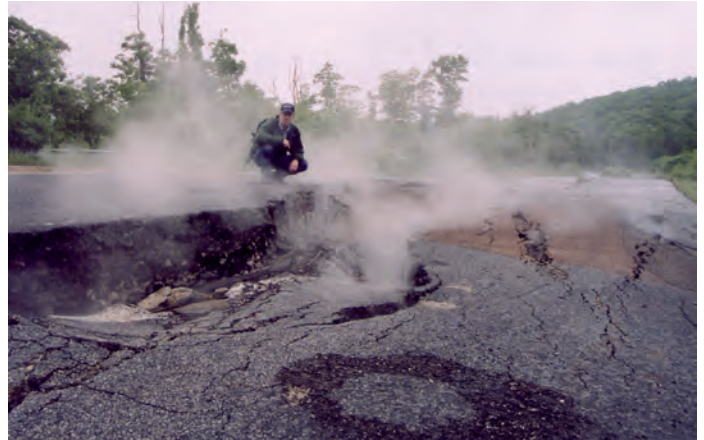
Figure 1. Emissions from the Centralia, Penn., underground coal fire; subsidence resulting from burning and subsequent collapse of coal pillars used as roof supports for mining tunnels under the town is also evident. Centralia, the largest and best known U.S. coal fire, has been burning since 1962 and has resulted in relocation of nearly all of the town's residents. Photograph by Janet Stracher.
