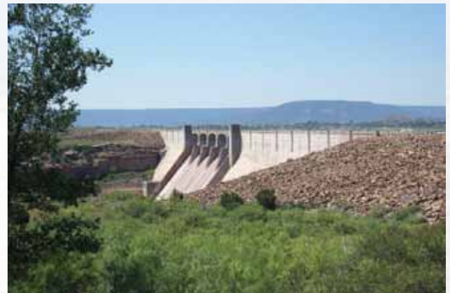
Conchas Dam near Tucumcari, New Mexico.
