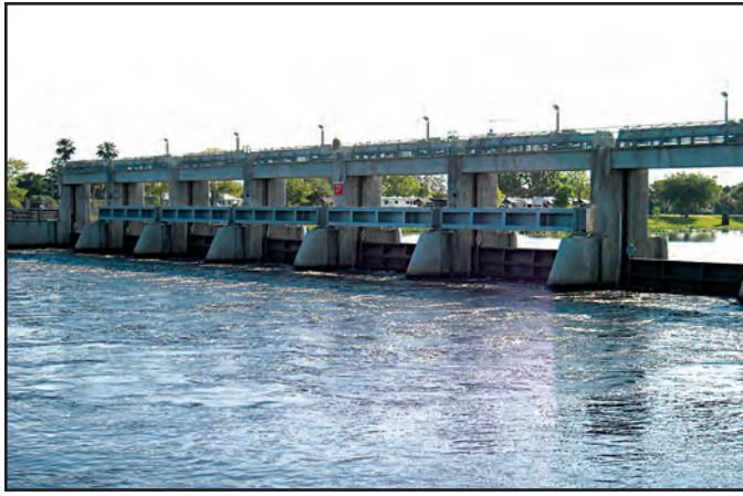
Figure 2. Control structure S-79 at Franklin Locks.
