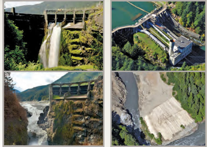
Glines Canyon (left) and the Elwha (right) dams before (top) and after (bottom) they were removed from the Elwha River. Photographs by John Gussman, private citizen.
