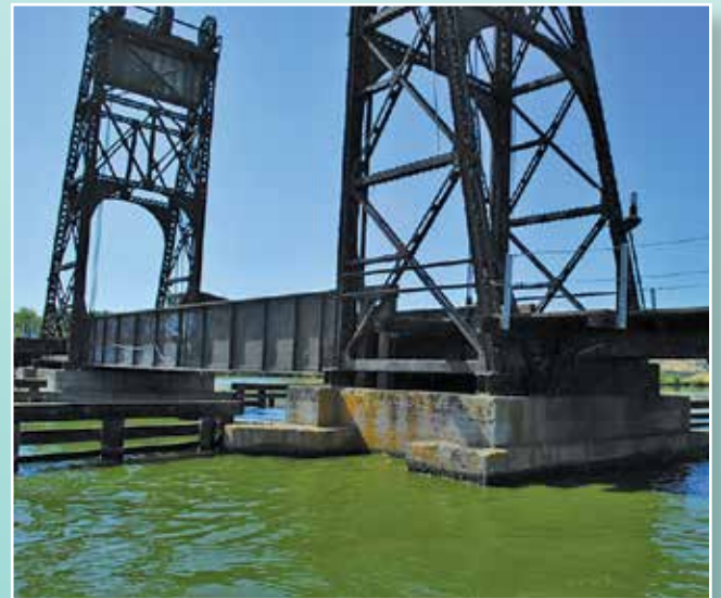
Water appears green near this railroad trestle in Lake Ewauna, Oregon, because of an algal bloom. (Photograph by C. Anderson, U.S. Geological Survey.)
