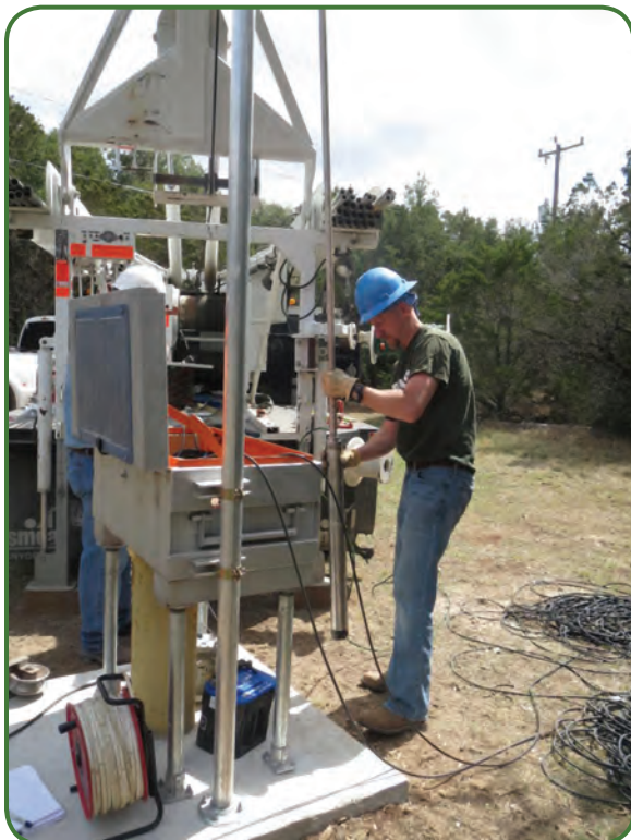
Pump hoist truck at the Shavano Park at Fawn Drive site.
