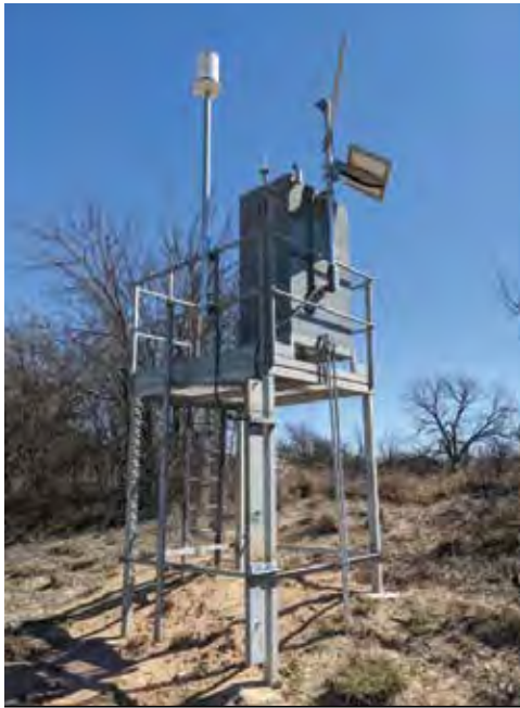
Figure 2. Continuous stream stage data are collected at the newly installed U.S. Geological Survey streamgage 08197970 Sabinal River at Utopia, Texas (photograph by Namjeong Choi, U.S. Geological Survey, February 26, 2020).
