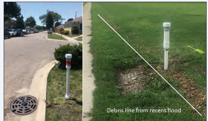
Figure 5. Low cost, water-level storm sensors installed in the Village of Harwood Heights, Illinois. Sensors were installed to monitor the height of water in the underground access structures or manholes and above the street. Photograph by William Selbig, U.S. Geological Survey.
