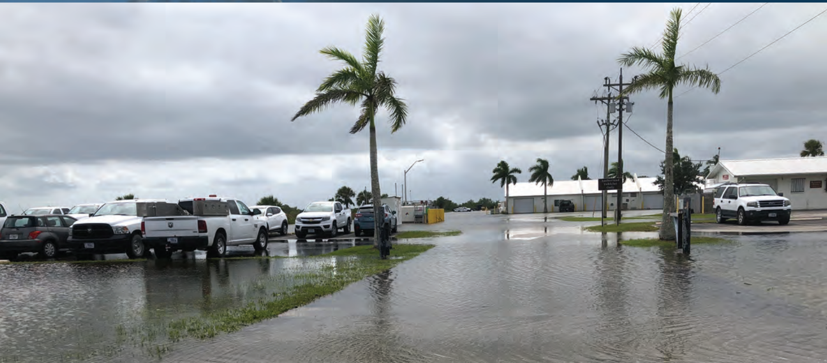
Figure 3. Flooding at maintenance complex behind the headquarters of Big Cypress National Preserve (BICY), Florida, on September 29, 2022, the day after Hurricane Ian's landfall. BICY headquarters is the western visitor center in figures 4 and 5. Photograph by National Park Service staff, BICY.
