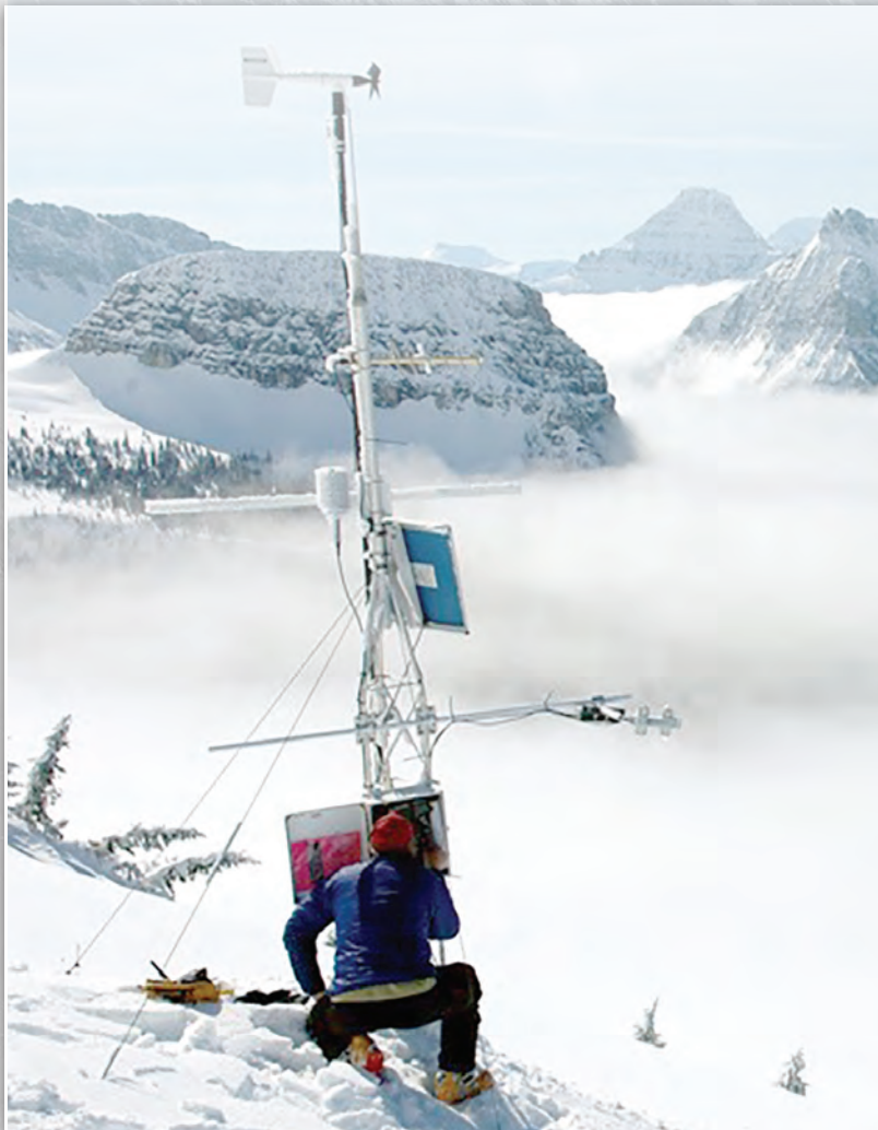
Figure 6. Photograph of the Garden Wall weather station, which is an upper elevation climate and weather monitoring station in Glacier National Park, Montana. Photograph by Erich Peitzsch, U.S. Geological Survey.
