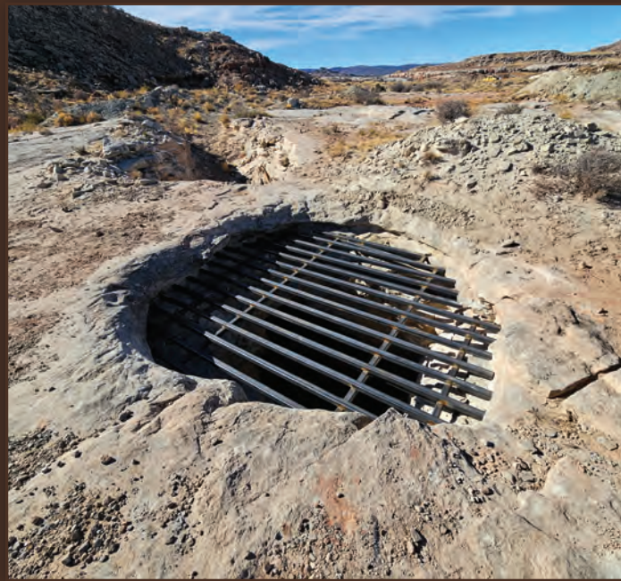
Figure 1. Photograph of a mine shaft in Utah that the U.S. Department of Energy’s Defense-Related Uranium Mines program safeguarded with a bat grate. The closure prevents human entry and wildlife entrapment while preserving habitat for bats. Photograph by Environmental Protection Services (Nevada).
